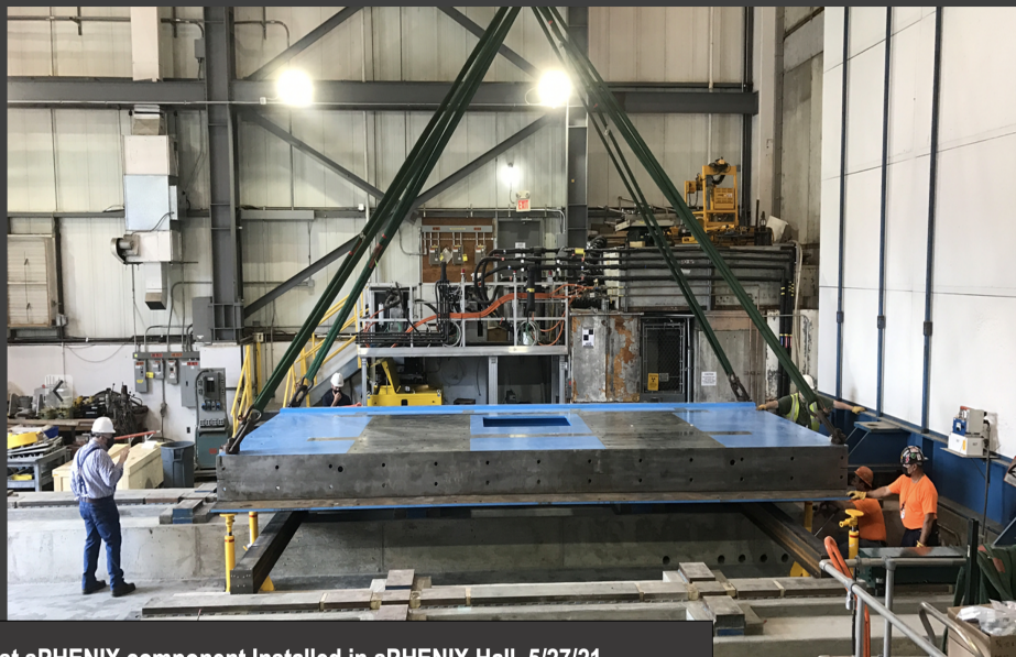
1st sPHENIX component Installed in sPHENIX Hall, 5/27/21
