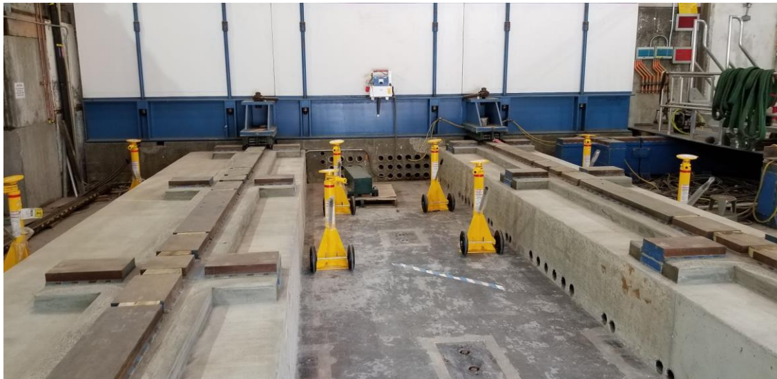
AH track upgrades complete
