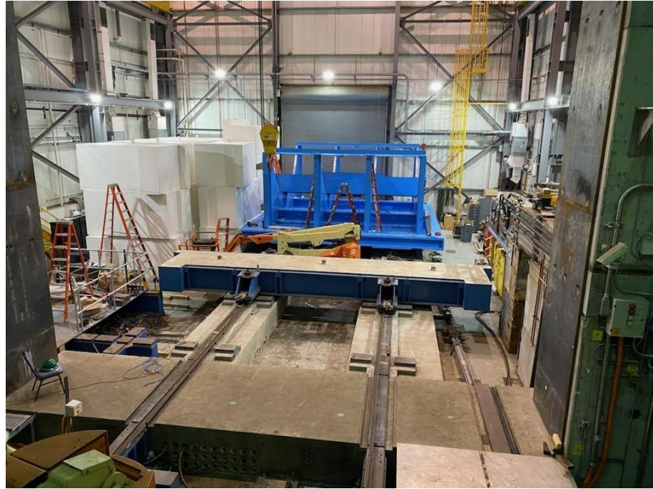
Looking at the sPHENIX cradle-base and dismantled shield wall blocks standing inside the IR
