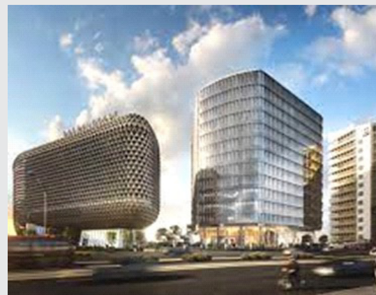
Rendering of the Bragg Centre under construction, Australia's first proton therapy center and the first center of its kind in the Southern Hemisphere.
