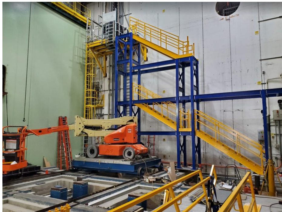
Completion of the IR west wall stairwell is a prerequisite for rolling sPHENIX into the IR. The west stairwell, which provides access to the sPHENIX L2 and L3 platforms and the cryogenics mezzanine, will be complete by 7/1.
