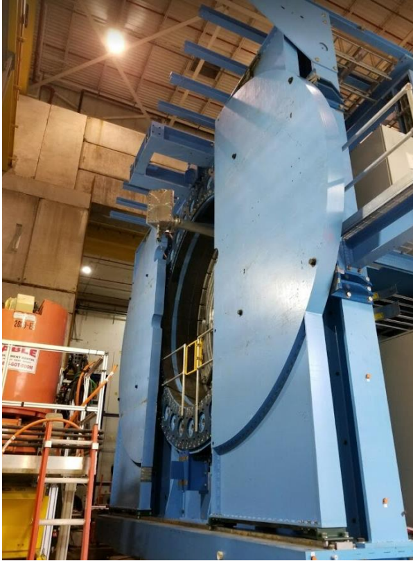
Initial installation of the south pole tip doors is complete. The north pole tip doors will be in place by 6/24. This will allow for the completion of the upper platform.
