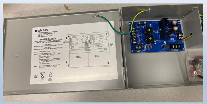
The intent is to provide batteries that meet / exceed code, which is 24h standby followed by 15m of alarm
