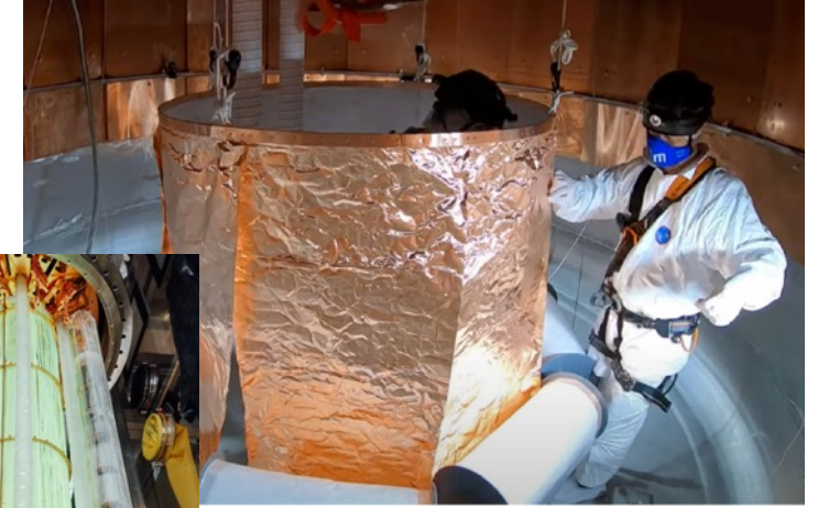
WaveLength-Shifting Reflector (WSLR) installed
