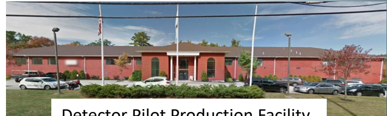
Detector Pilot Production Facility
