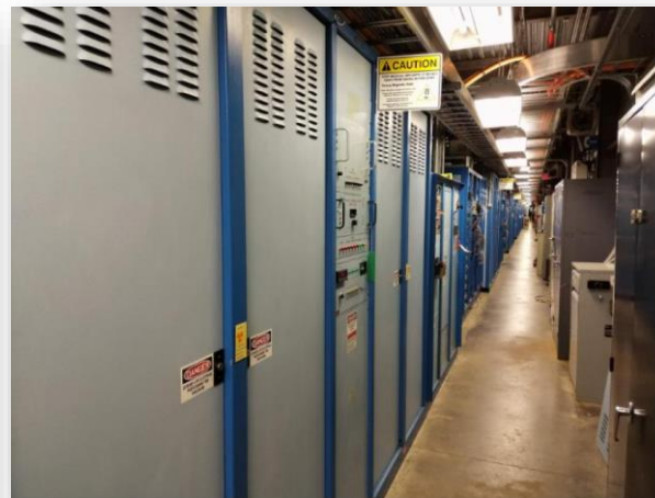
418 Klystrons for 52.25 Cryomodules
