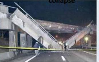
Dec. 2005 , 45 years after the construction Pennsylvania. Rebar corrosion because of ant freezing agent
