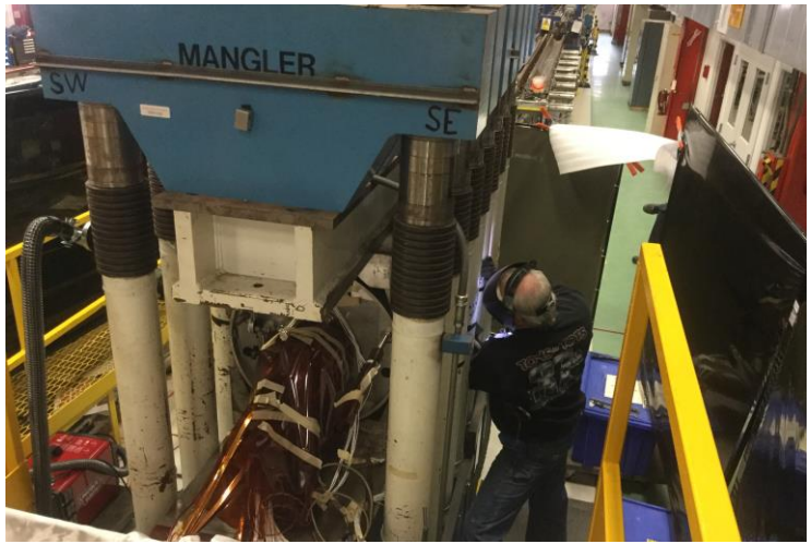
The stich welding under press load
