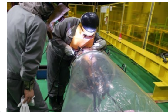
End ring welding
