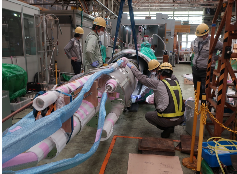
Preparation of Leak Check
