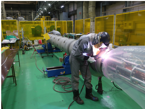
End Dome Welding
