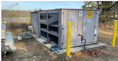
Removal of existing 1004B AC unit in preparation of new unit arrival
