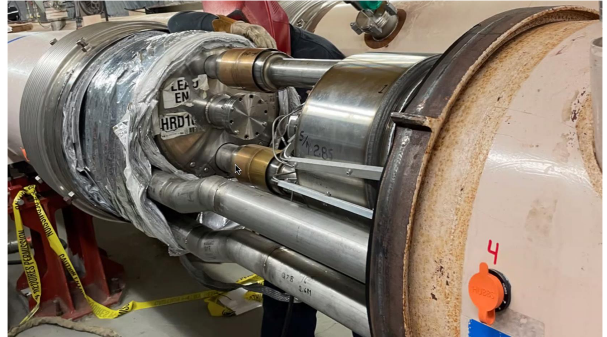
Utility lines completed and welded (10 o'clock side)
