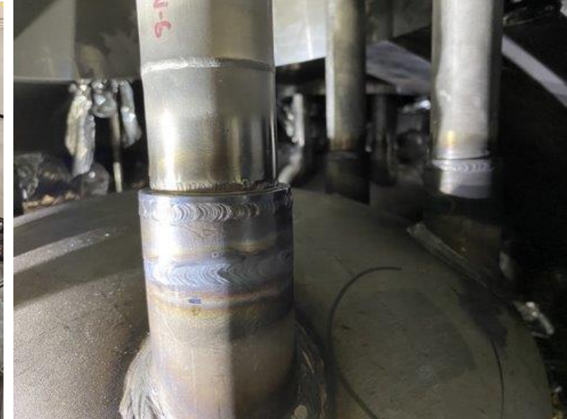
Feedthrough, new feedthrough tube and bellows installed
