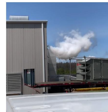
Helium venting at Bldg. 1004B
