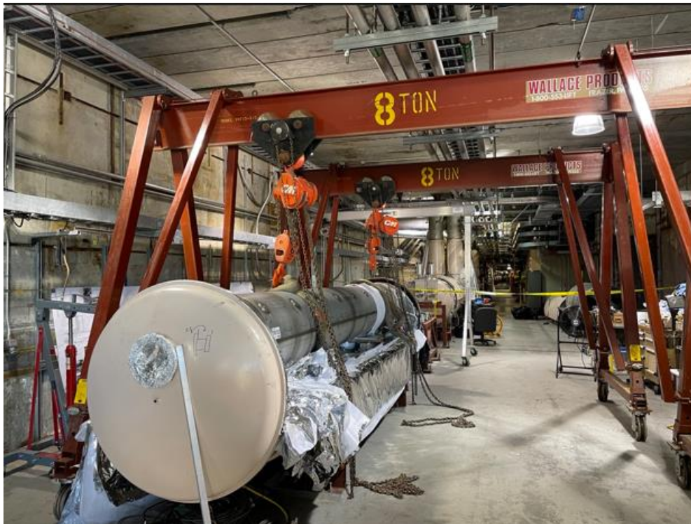
DX magnet in tunnel prior to removal (IR 4 region)
