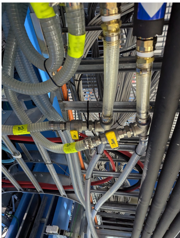
MVTX Temporary T Solution sharing cooling between staves and electronics.
