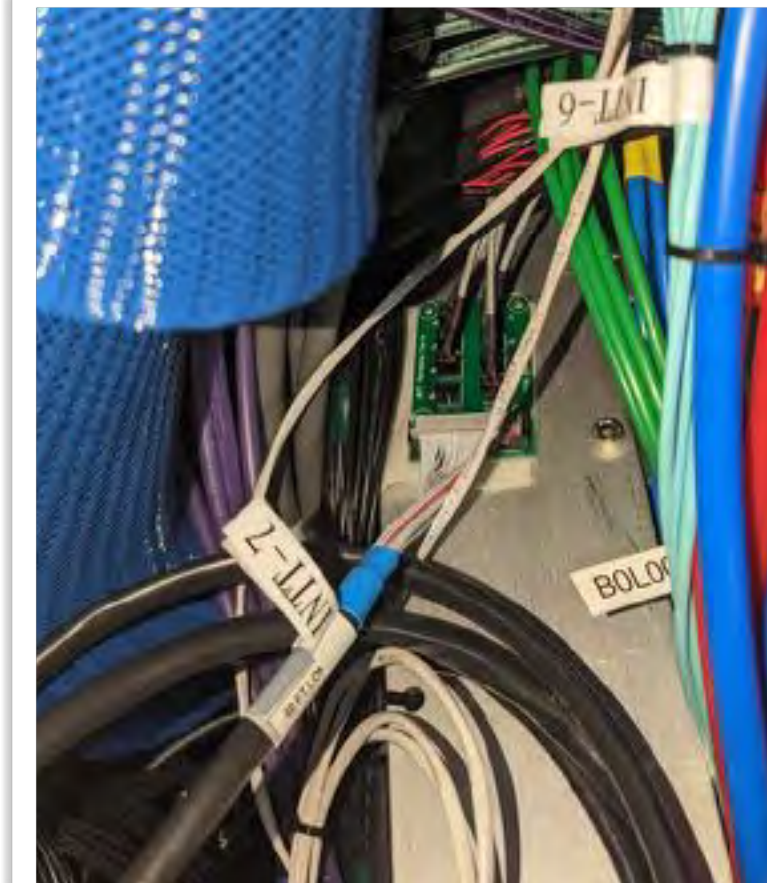
Thermistors 112 + 16 = 128 cables
