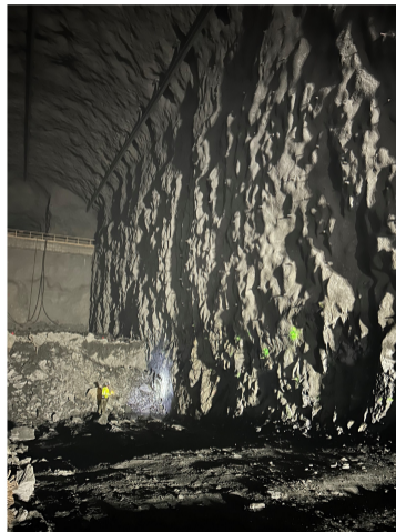
Performing geological survey
