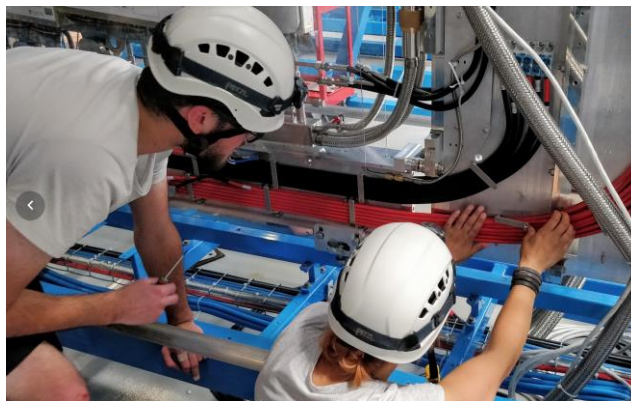
Installing bias cables.
