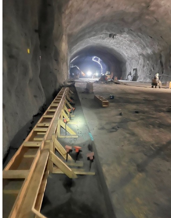
Central utility cavern
