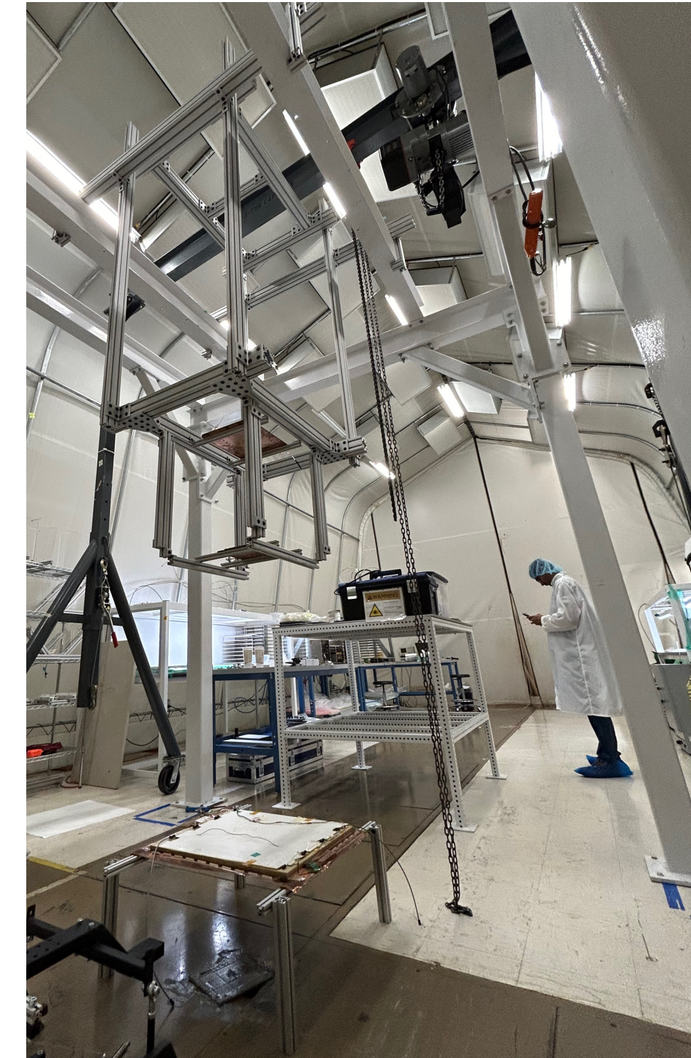
Installation and alignment of CRT tracking stations
