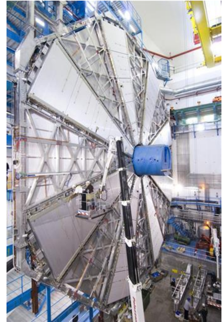
Big Wheel (endcap) built in the US, installation in ATLAS
