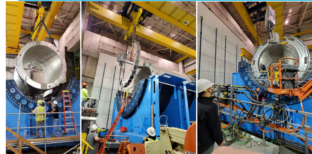
Photos of Magnet Installation from sPHENIX Experiment
