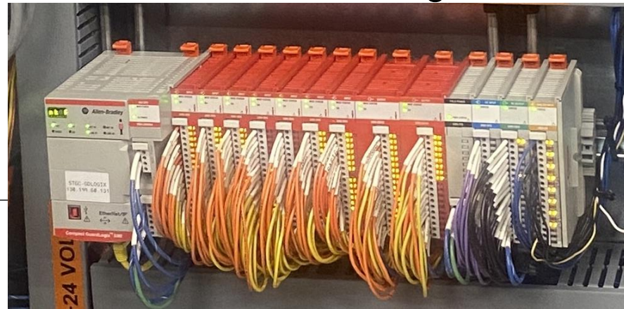
Allen-Bradley GuardLogix safety PLC And Safety IO cards
