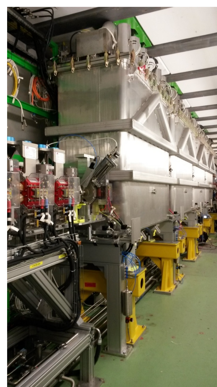
Picture 1: The view inside the HIE tunnel.
