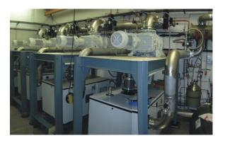
2 K refrigerator providing ~120 W (SULZER TCF 100/2K L/R, 1982)
