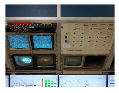
Personnel and machine safety interlock, monitoring cryo plant
