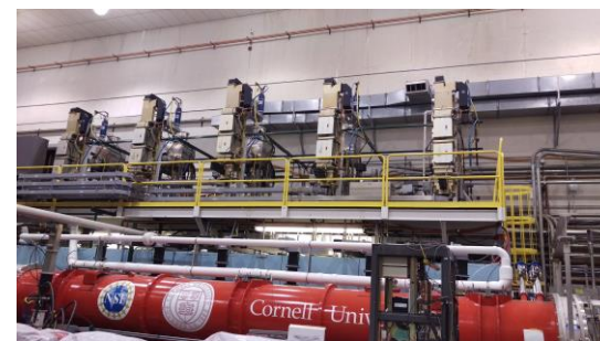
Klystron Platform 59 Hz vibrations coupled in through waveguide suspended from platform.
