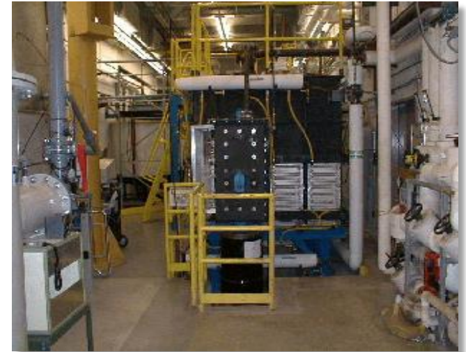
VSL DM1200 HLW Pilot Melter System
