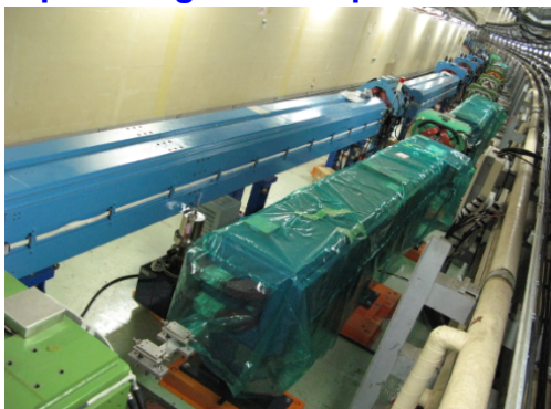
TiN coated beam pipe with antechambers
