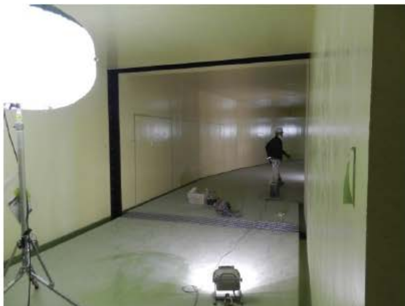
Inside DR tunnel
