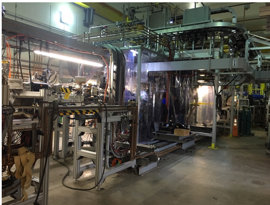
Fig. H. 25. All CeC equipment, including the modulator, FEL and the kicker, has been removed from the common section at IP2. Only quadrupole support stands and cable trays remain on place.
