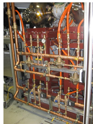
Fig. H.8. Left: Phase I (low energy) beamline with solenoids (black) and vacuum pipes during installation; Right: Water-cooling distribution system for 500 MHz (seen on the background) and 113 MHz system
