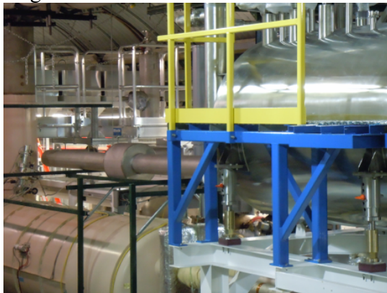
Fig. H.7. Left: The CeC's quiet helium source (top-right) is installed at IP2 above RHIC magnets. The photo was taken when the first of two LiHe transfer lines to 113 MHz gun is being installed. Right: The solenoids on their supports installed in the IP2.
