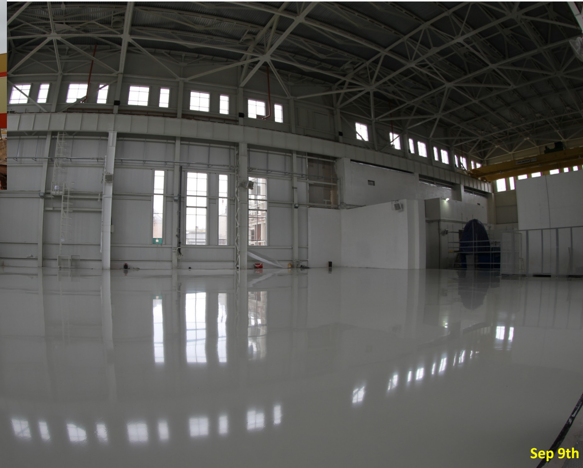
Epoxy floor finish ready in the MPD Hall
